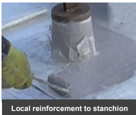
Local reinforcement to stanchion
