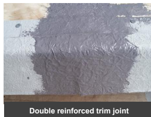
Double reinforced trim joint
