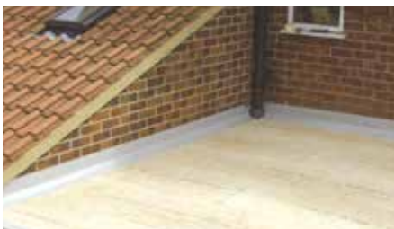
Any other protrusions such as pipes, skylights or other potential weakspots should also be laminated around/over at this point. Any joints between trim lengths are bandaged over.
